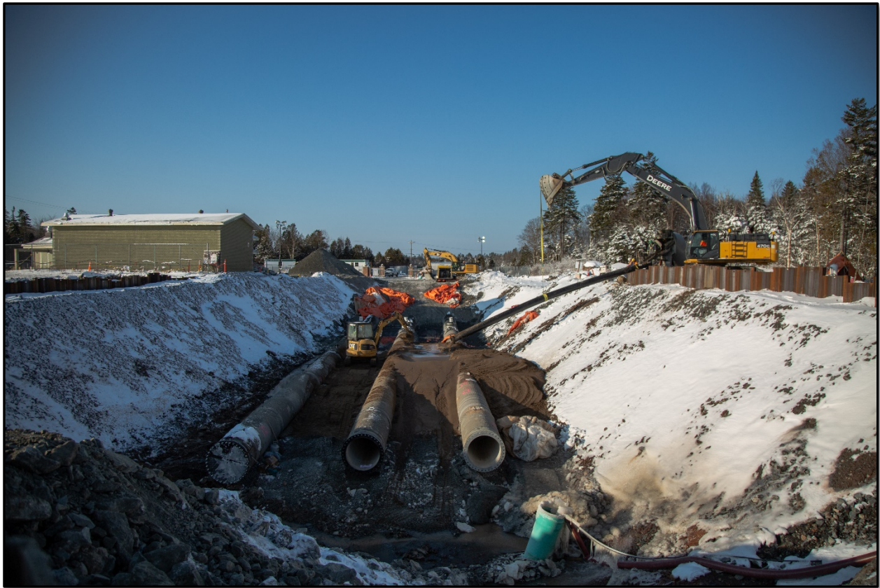
New Raw Water Intake Installation – Latimer Lake Winter 2019
