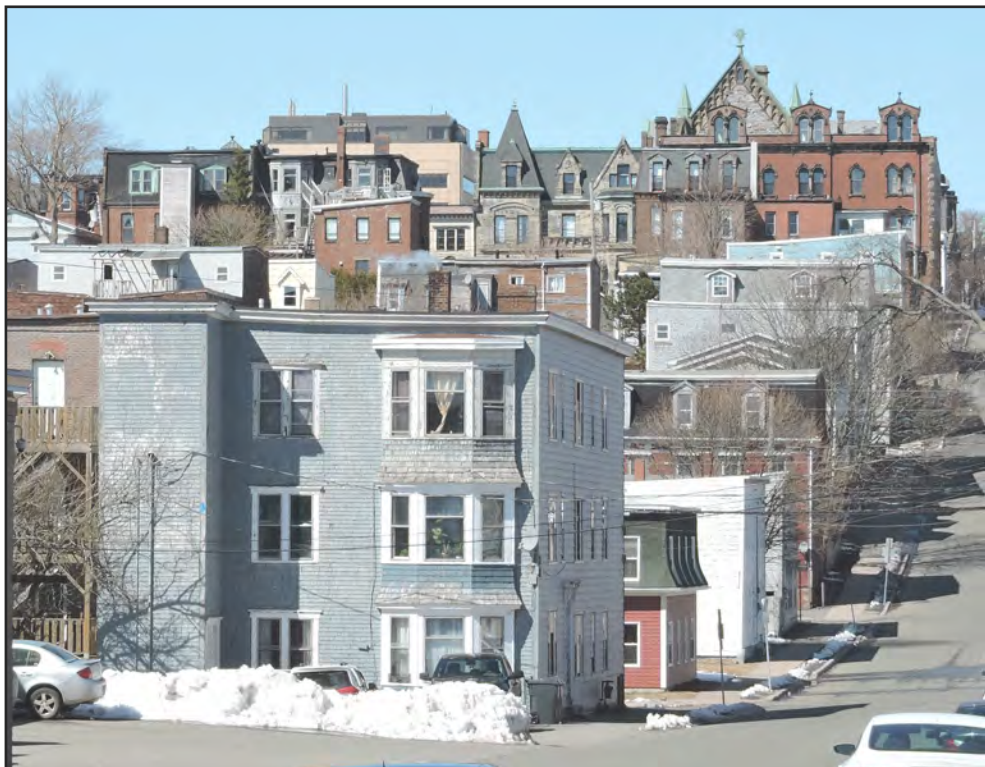
SOUTH END - WOOD BUILDINGS AND LARGER MASONRY BUILDINGS SET ON A HILL
