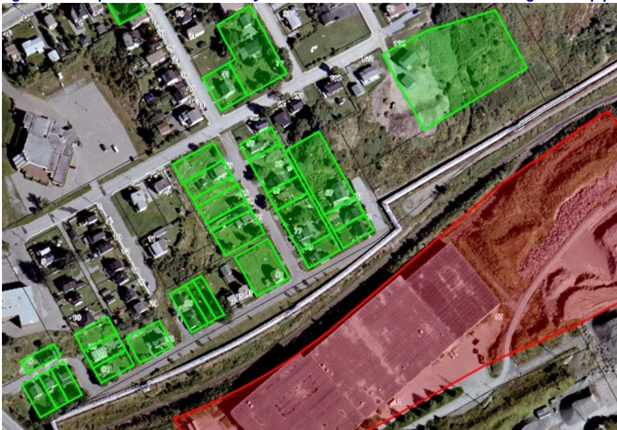
Figure 2.4: Properties on Pleasant City St. and River Ave. demolished following butane pipe leak in 2019
