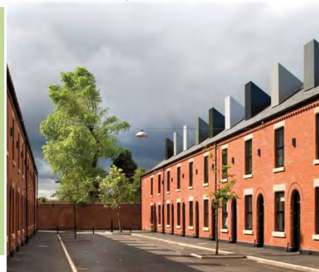
CHIMNEY POT PARK, SALFORD, U.K.
