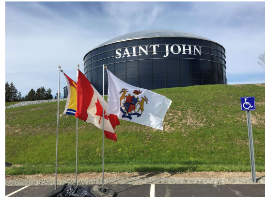
The Loch Lomond Drinking Water Treatment Facility tanks hold up to 33 million litres of clean water.
