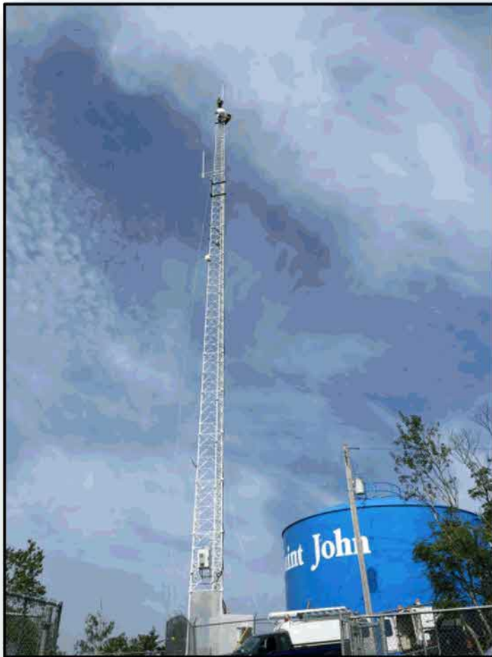
Rockwood Park Reservoir & Communications Tower SCADA Communications Repair July 2015
