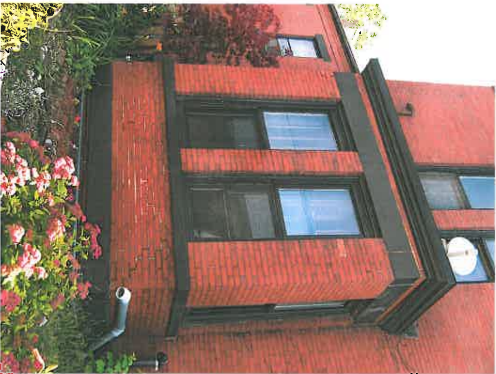
Box Bay Window - Repoint
